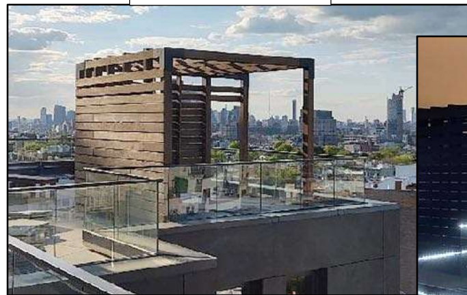
Installed On Client's Site
