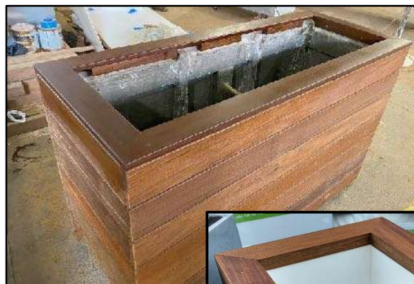
IPE Clad Planter Over Our Fiberglass Liner
