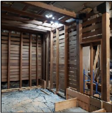
Constructed in Our Workshop
