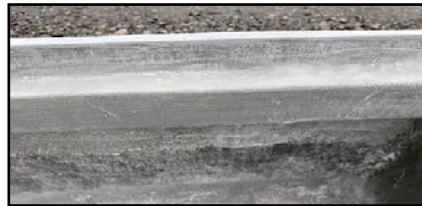
Fiberglass Board covered with fiberglass supports perimeter of planter
