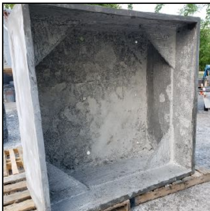
Corner Support Structure
